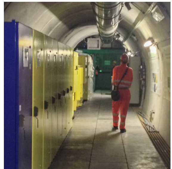
Cross passage linking the east and west bores Photo R Werner
