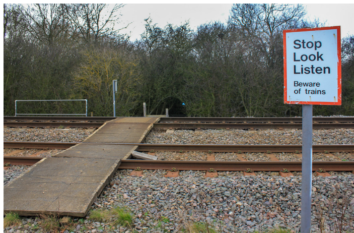
User-worked crossing on the Stratford to Birmingham line near Newnham, Warwickshire, UK (photo David P Howard)
