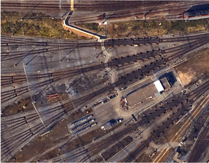
Five principal tracks and their retarders (track brakes) lead to Lausanne marshalling yard's 38 destination tracks. Photo copyright Google Earth, used with permission.
