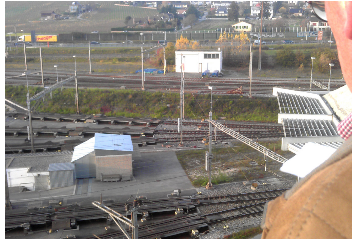
Dieter Kaupp, former lead developer of hump-yard control for Siemens in Switzerland, presented the Lausanne yard's five retarders. The main-line tracks of Denges junction are in the far background. Photo George Raymond.
