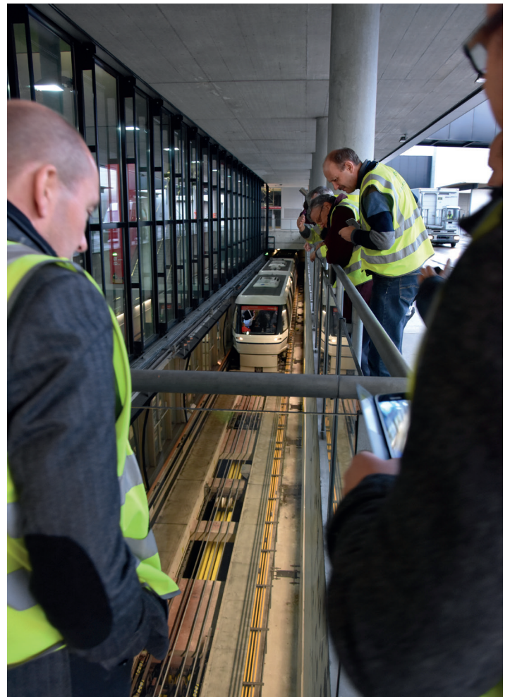
During the Skymetro's 2009-2010 partial shutdown, the airport's Gate E34 closed for six months for construction of this opening, which let cranes lower three more cars into the Terminal E station.
