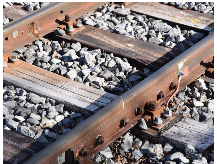
Diagonally cut Insulated Rail Joint.
