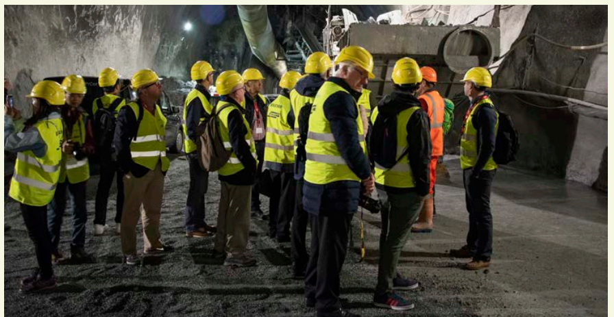
Members inspect the construction of the new Albula tunnel.
