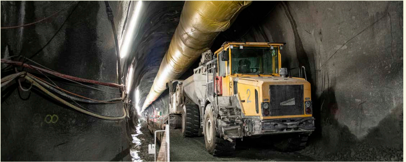
Inside the RhB's new Albula tunnel.
