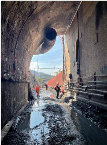
Massive civil works were performed for example blasting, diamond cutting rock and concrete, pressure washing the arch
