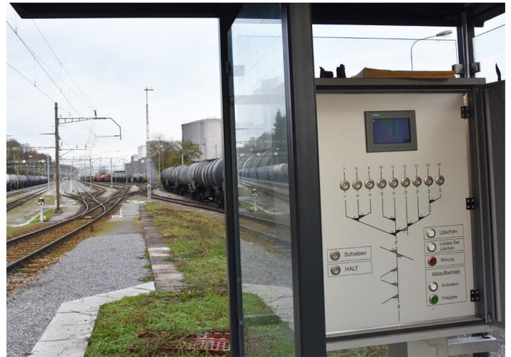
The re-signalled, nine-track Aufhafen hump in 2019 and its new local control panel, which an operator can use wearing gloves. Photo George Raymond.
