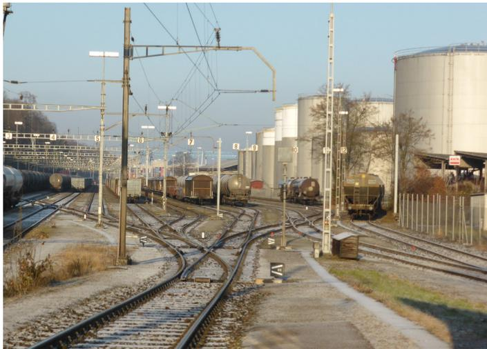
The nine-track Auhausen hump yard in 2013, before re-signalling. The project removed the connection between tracks 4 and 5 and renumbered all tracks. Photo Bruno Huber.
